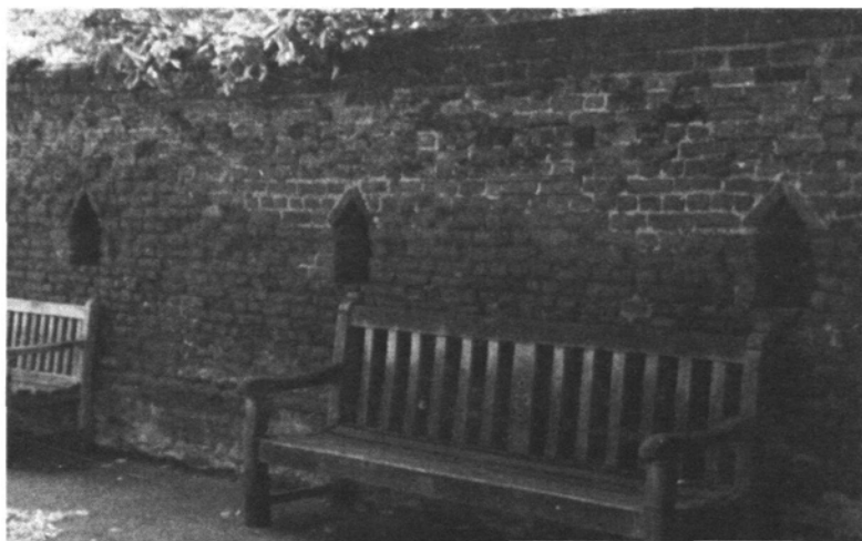
Three of the six bee boles in an east-facing brick wall, Cathedral Close, Canterbury (287). (Photo.: David A. Smith, 1984)
