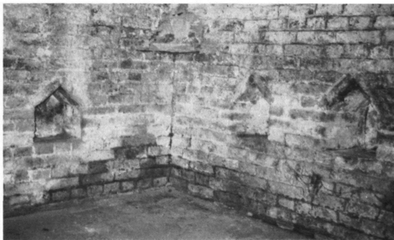
Three of nine recesses in a cellar, St. Stephen's, Canterbury (375c), probably built in 1490 and used for the winter storage of bees. There are 20 bee boles in the garden of this house. (Photo.: Paul Campbell, 1986)
