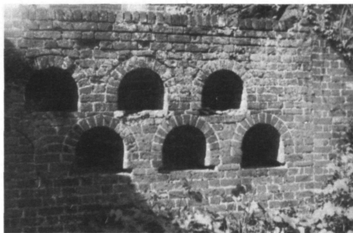
A two-tier set of Tudor bee boles at Plaxtol (248); slots for separate wooden bases are visible in the lower row. (Source: V.F. Desborough, Arch. Cant. , lxi (1955), 90-5)
